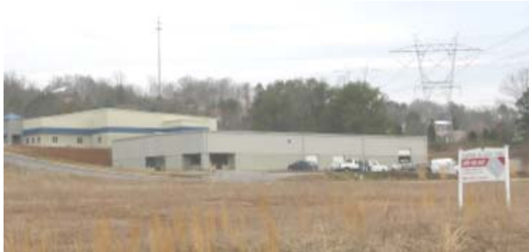
The Topside Business Park on SR 333 is generally in the vicinity of commercial uses.
